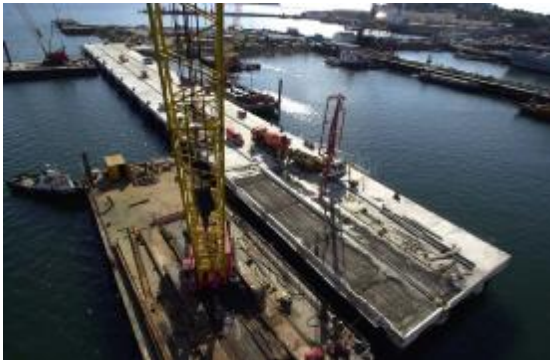
Construction Works at Queens Wharf -
