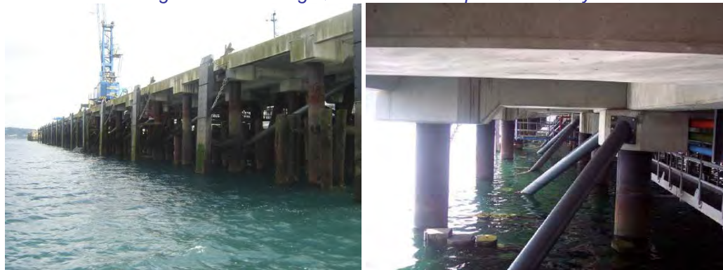
Figure 2-11 Existing Queens Wharf's Open Piled Quay
